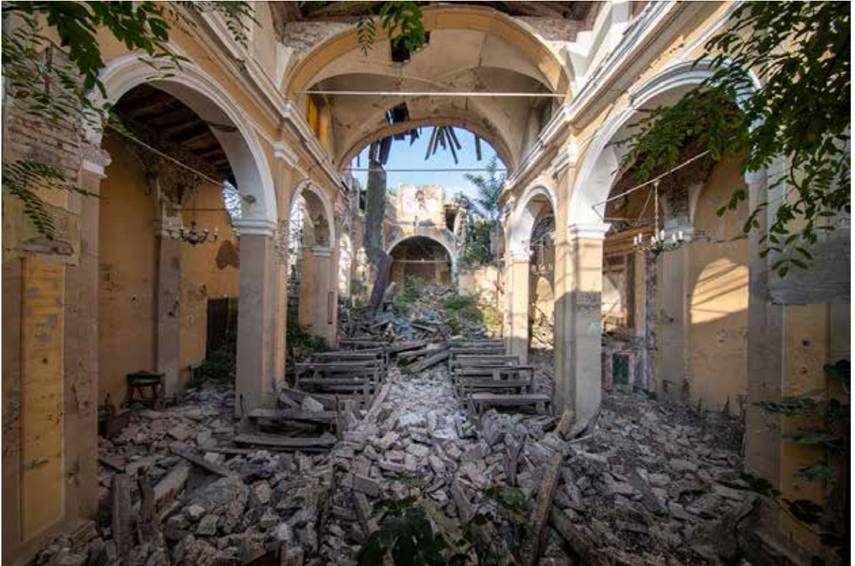
Crumbling to Pieces (362)
